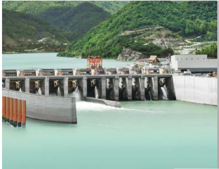
The ANDRITZ turbines have a very fish-friendly design.
